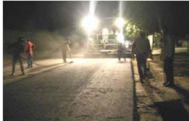
Night crews work on Shash Darak Road in Kabul City.
