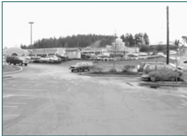
Action Team photo Freeland, in unincorporated Island County, has stormwater issues similar to those in urban areas.
