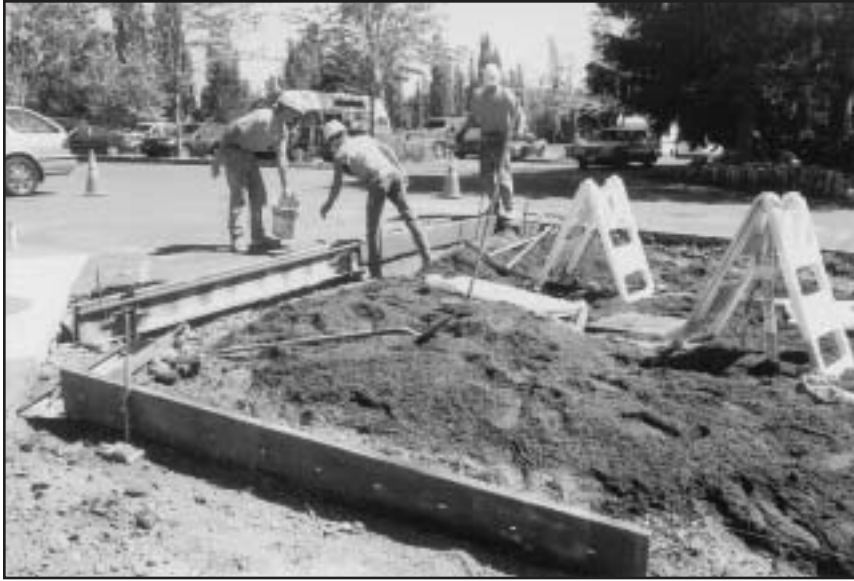
Rain garden construction site at Bloedel Donovan Park.
