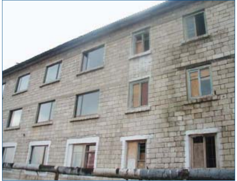
Forty public buildings underwent energy efficiency weatherization in Moldova
