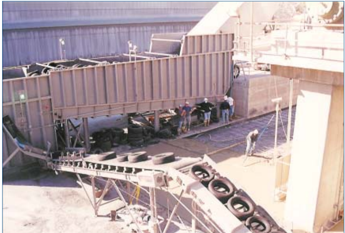
Central American cement manufacturers visited this cement plant in California that burns used tires for fuel
