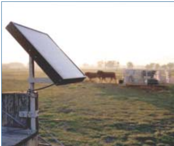
Solar panel powering an electric fence
