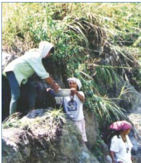
Villagers passing sand and gravel to the construction site
