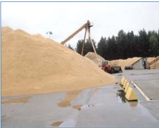
Gethal Amazonas converts the wood waste to power using a 5.5 mW boiler and a high-pressure steam turbine generator
