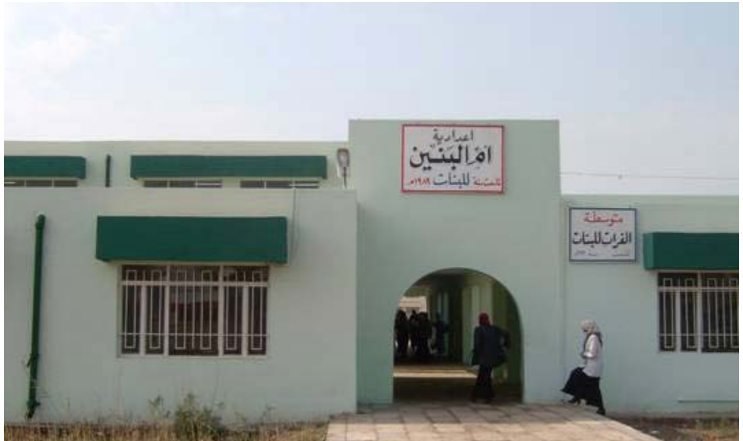
Photograph of Um Al-Banin School in Al Hillah. This school was rehabilitated by USAID funds through a contract with Creative Associates International, Inc. (Creative). (Photograph taken on December 3, 2003)
