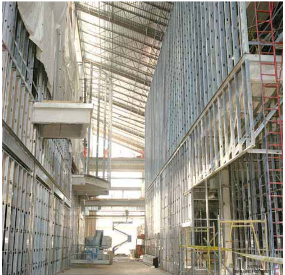
The Metropolis Center atrium awaits drywall installation.
