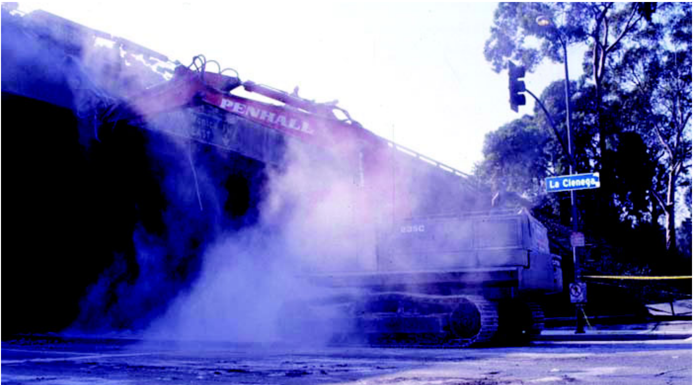
Figure 14. Demolition of I-10 at La Cienga Boulevard
