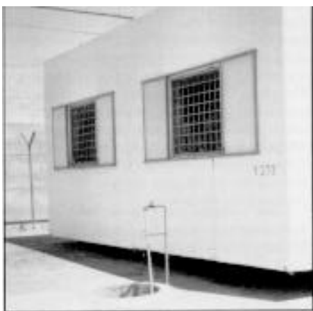
Isolation building, military prison camp Ketsiot.
