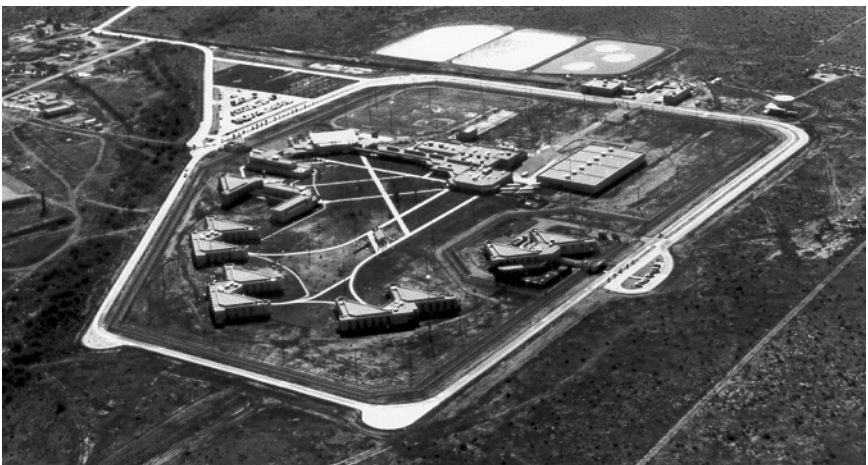
Federal Correctional Institution, Phoenix, Arizona.
