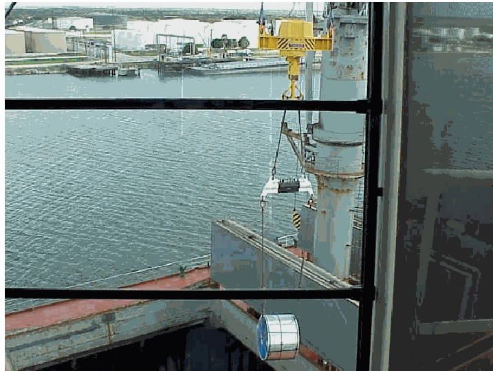
New crane at the Port of Brownsville
