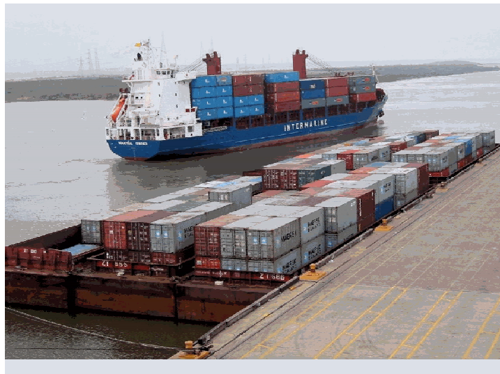
Hopper barges at the Port of Brownsville
