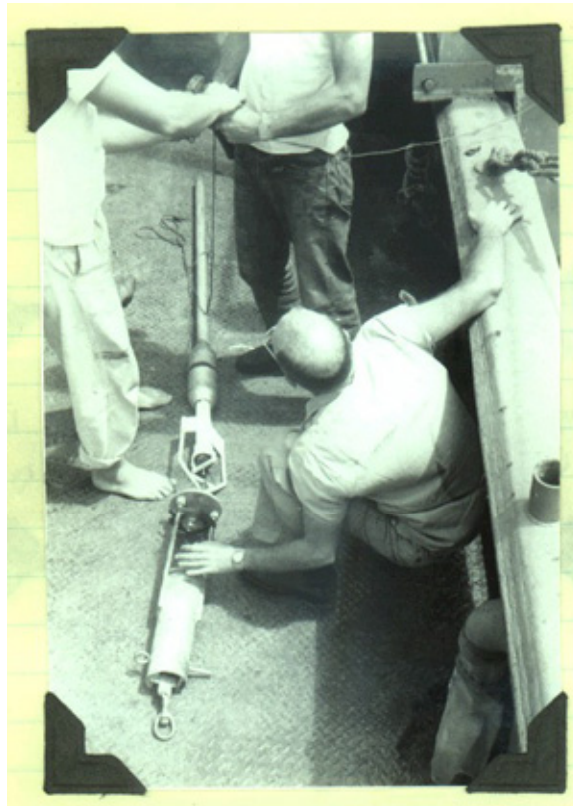
Getting the ball breaker and coring device ready for a lowering.
