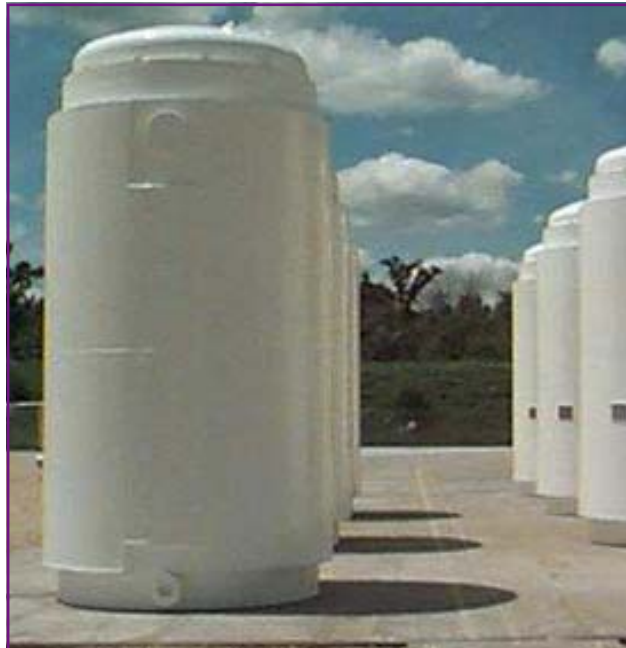
Onsite dry cask storage
