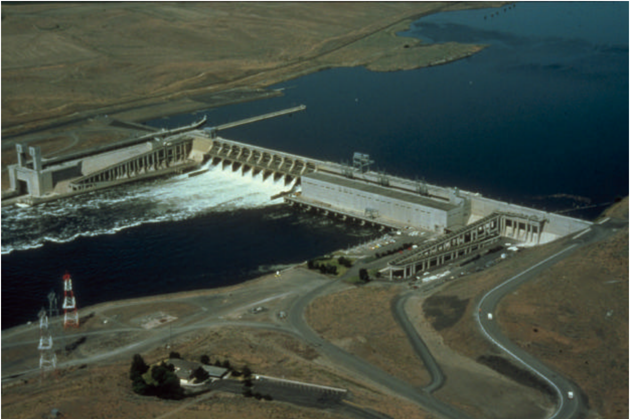
Figure 2-4. Ice Harbor Dam
