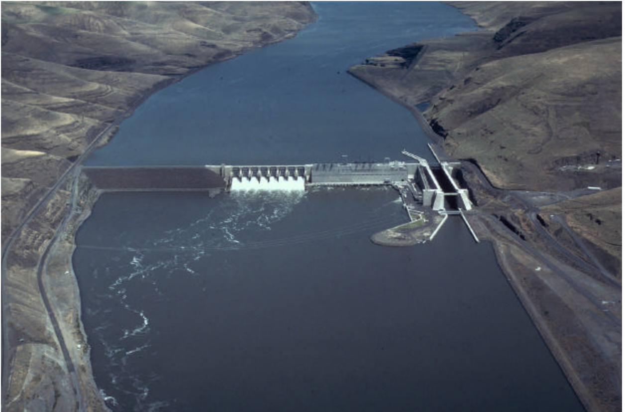
Figure 2-2. Little Goose Dam
