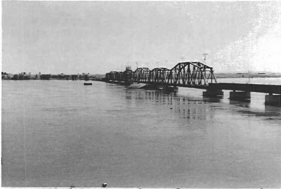
BARGE STUCK UNDER UPRR BRIDGE. 28 JUNE 1974
