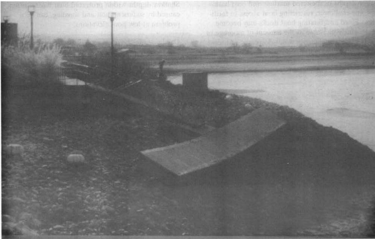
Figure 2-4. Typical Effects of Extreme Drawdown at Run-of-River Reservoirs (Lower Granite)
