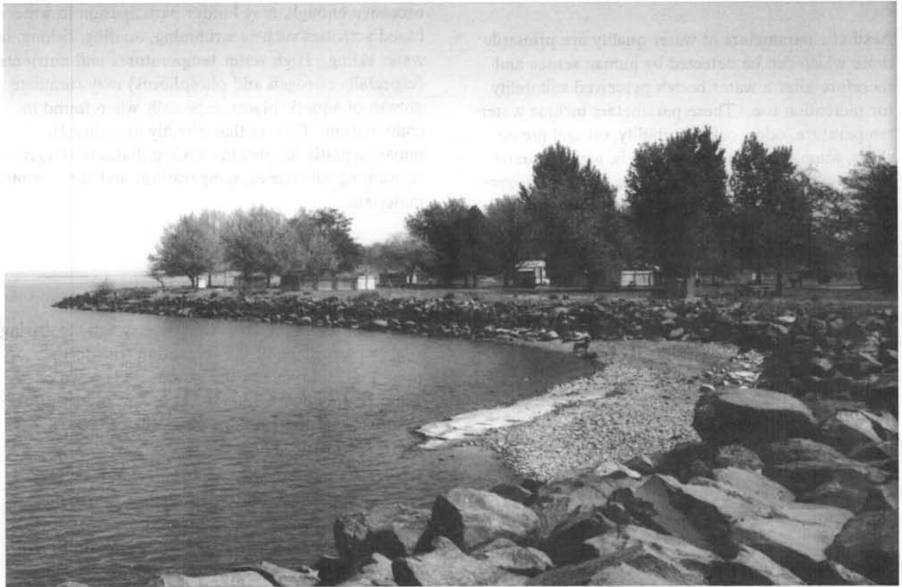
Figure 2-7. Bank Protection is Needed to Prevent Shoreline Erosion at Many Recreation Sites
