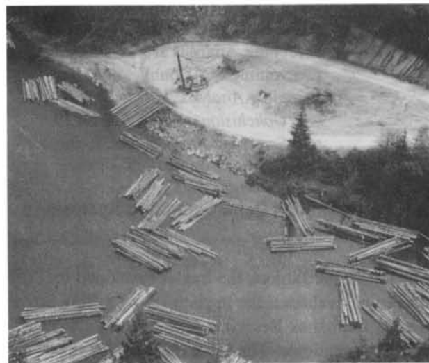
Figure 3-3. Dworshak Dam Log Dump
