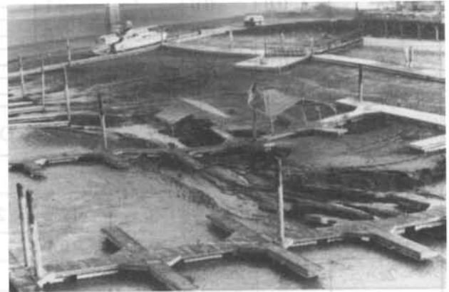
Figure 3-4. Damage to Red Wolf Marina in the Lower Granite Pool during March 1992 Drawdown Test
