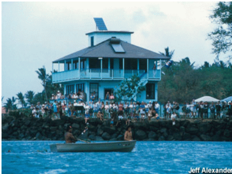
Spectators watch from the shore as nets were cast for the fishing demonstration. Behind the audience stands the Maui Sanctuary office, a volunteer-renovated building that was once home to the National Weather Service. (photo: Jeff Alexander)
