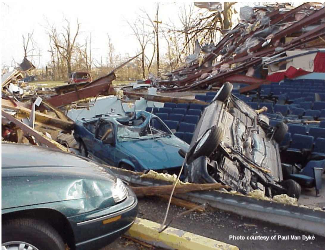
Van Wert, OH Tornado Damage: As a result of NWS' timely and accurate warning, no lives were lost when a tornado destroyed this movie theater.
