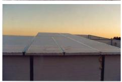
3. The roof is also constructed of foam panels that are held in place by aluminum channels. Once covered with Grancrete, the roof becomes an integral, water-tight part of the home.
