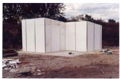
2. Lightweight aluminum channels also are used at the corners and between every 4-foot by 8-foot panel to hold them in position during spraying. From start to finish, all of the foam panels for the walls and roof can be installed and ready to be covered by Grancrete cement in just a few hours.
