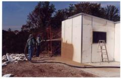
4. The window and door openings are cut out of the foam, and the frames installed. Conduit and pipes for electrical and plumbing utilities can be attached to the foam and then sprayed over with Grancrete to conceal and protect them.
