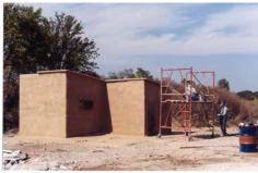
5. Both the exterior and interior of the walls and roof are sprayed to a thickness of about one-half inch. Grancrete is sprayed around the windows and door frames to ensure a weather-proof seal.
