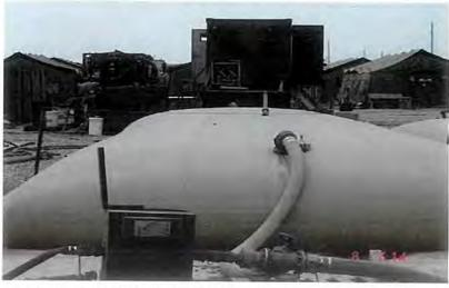
Figure D-17 (U): ROWPU Water Bladder
