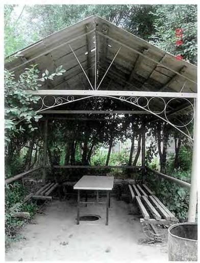
Figure D-6 (U): Gazebo near CI/FP Bldg with Asbestos Tiles
