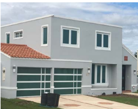
Figure 6. Fixed and operable window assemblies at a home performed without failure.
