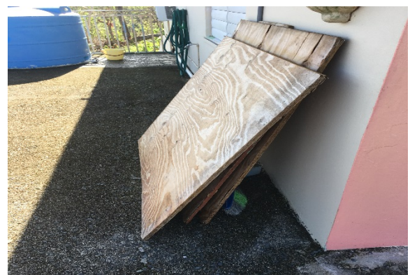
Figure 14. Top, metal louverie window that was protected from wind-borne debris by wood panels, bottom, during Hurricanes Irma and Maria.
