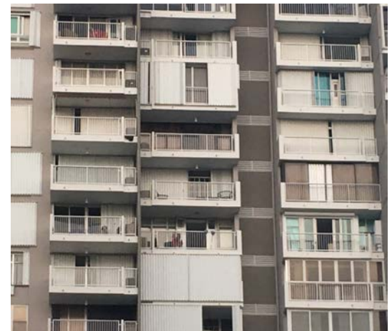
Figure 11. A high-rise residential tower where approximately 85% of units have a form of shutter or impact-resistant system in place that was installed as a retrofit.
