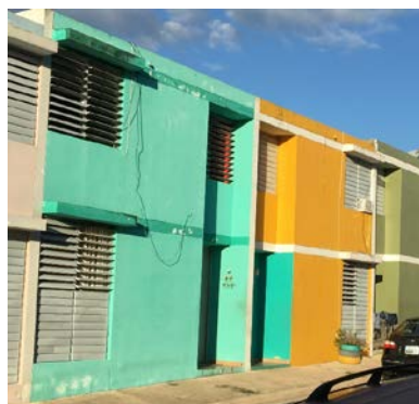
Figure 3. New secured housing units with metal jalousie openings.
