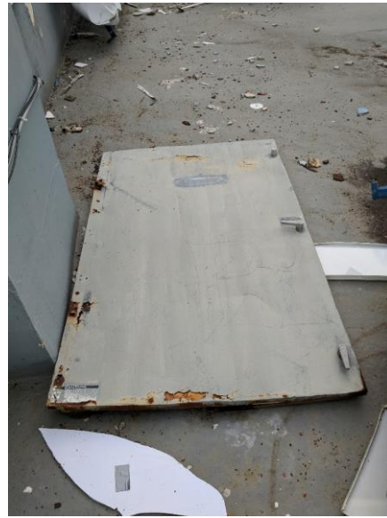
Figure 4. Left, HVAC unit with blown-off access panel; right, a blown-off filter access panel.
