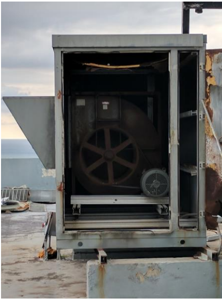
Figure 4. Left, HVAC unit with blown-off access panel; right, a blown-off filter access panel.
