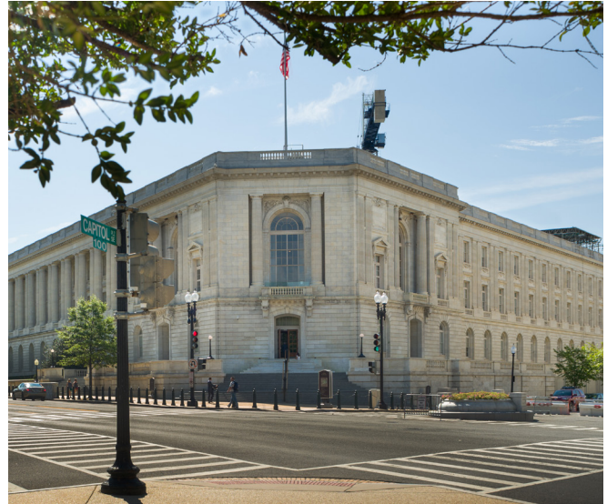
Work during the initial phase of the Cannon Renewal Project includes updating building utilities, primarily in the basement and the moat area of the courtyard.
