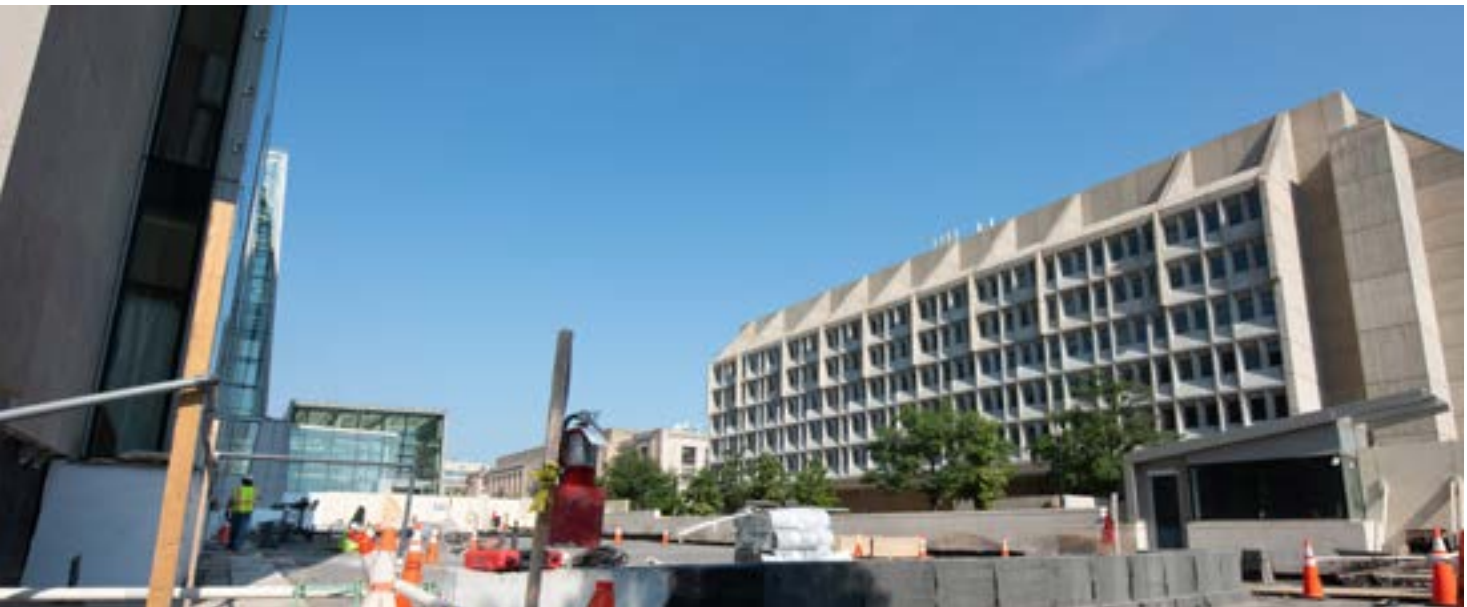
Exterior construction of the O'Neill Building. Photo by Phi Nguyen.
