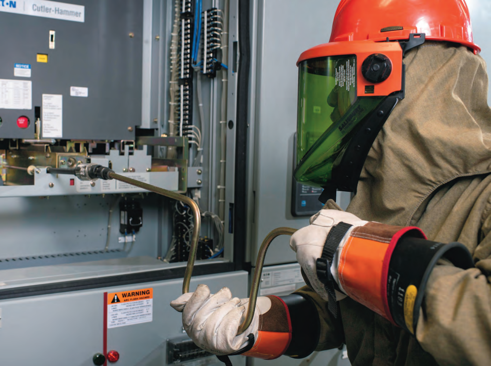
High-voltage electrician Da'suan Mason follows precise procedures and wears a fireproof 40 cal arc flash suit while performing regular preventive maintenance on a 15,000 volt circuit. Photo by Dewitt Roseborough
