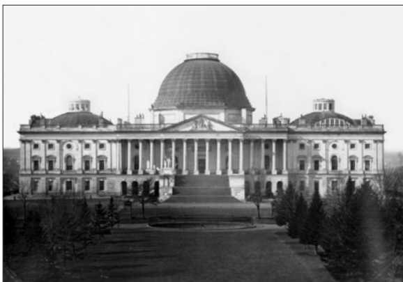
The U.S. Capitol, 1846; the Supreme Court was located in the Senate wing, on ground level at right
