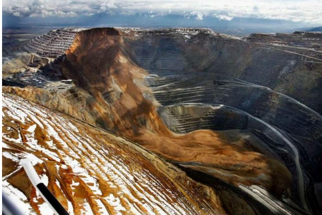
Bingham Canyon Mine Landslide, April 10, 2013
