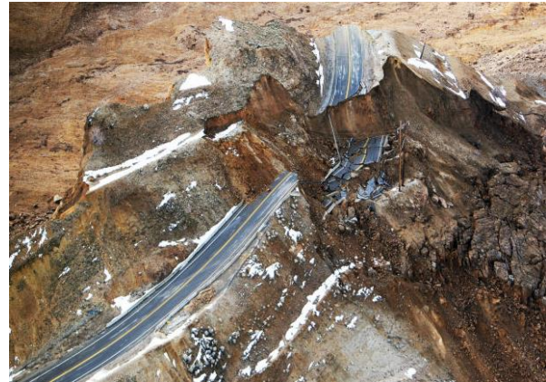
Bingham Canyon Mine Landslide, April 10, 2013
