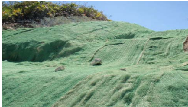
Terraces and geotextile
