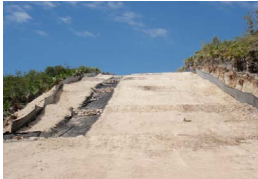
Longitudinal/transversal furrows and velocity dissipation devices
