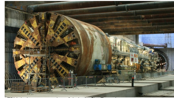
TBM during construction of Leipzig City Tunnel
