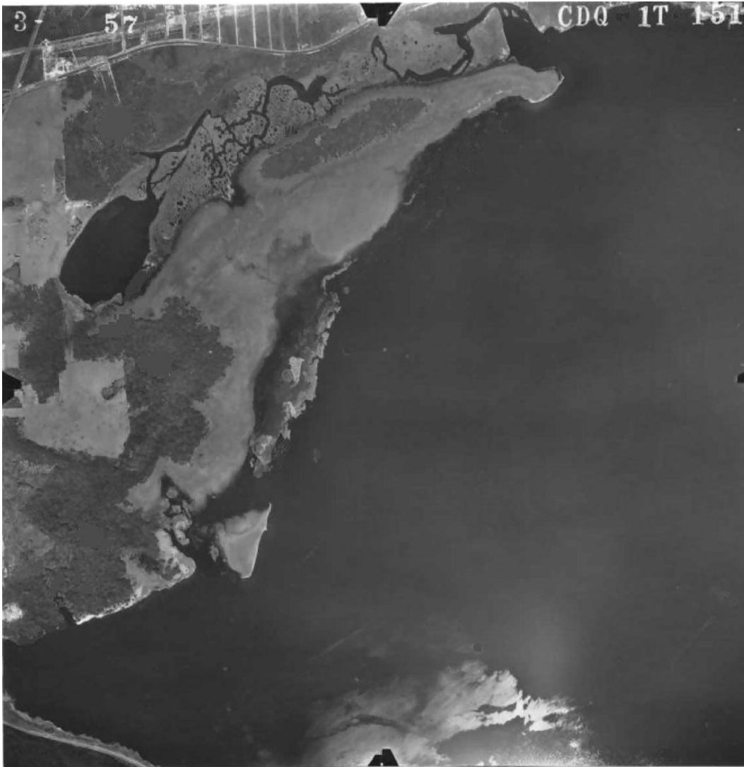
Figure 11. Aerial photograph,1957, DeBary Bayou and Lake Monroe, stage 0.84 ft. Image prior to I-4 construction. Image not to scale in this reproduction.
