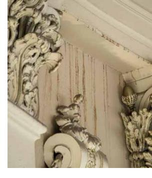
Water infiltration has led to leaking and staining in the Rotunda.
