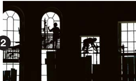
2 Workers prepare Rotunda for safety canopy - April 2014.
