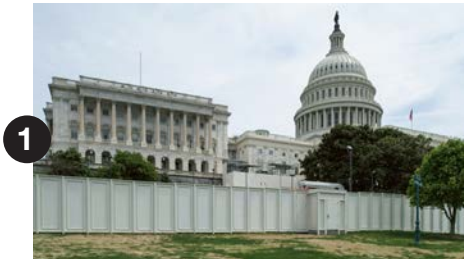
1 Construction staging area on the West Front - March 2014.
