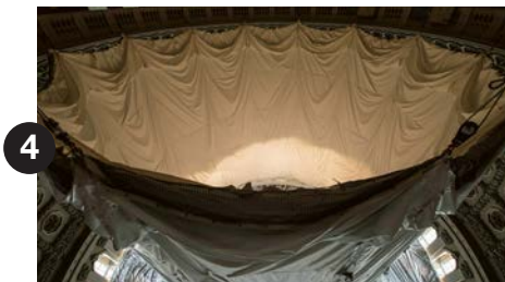
4 Safety canopy rising in Rotunda - April 2014.
