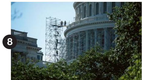
Scaffold access tower constructed on roof - July 2014.
