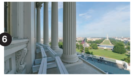
6 Scaffolding preparations on Peristyle of Dome - June 2014.
