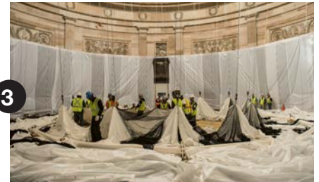
3 Safety canopy prepares to rise in Rotunda - April 2014.
