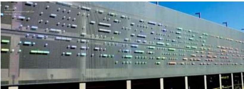
"Horizon" on the side of the parking garage behind the administration building cost $285,000.
