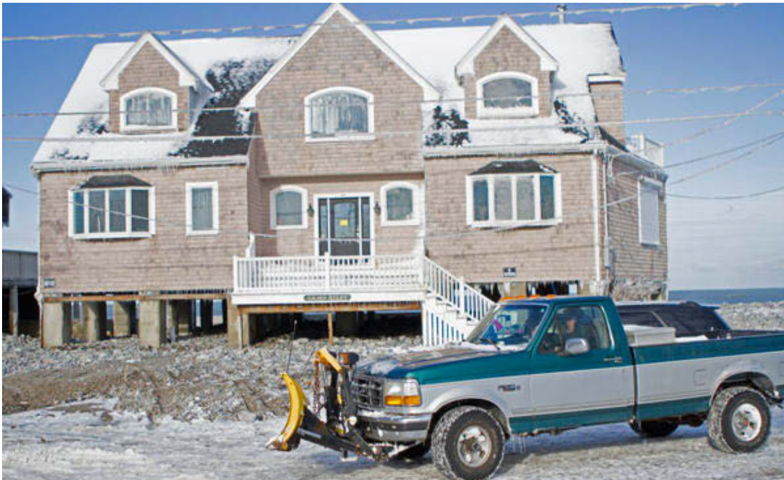
The million dollar mansion at 48 Ocean Drive in Scituate, Massachusetts, received $180,000 this year from the National Flood Insurance Program, which is $24 billion in debt.
