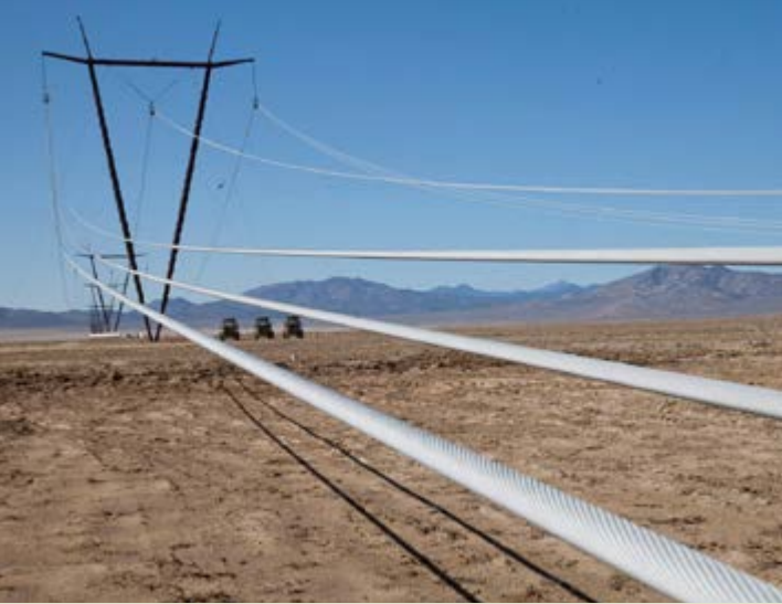
Construction of the One-Nevada Transmission Line
