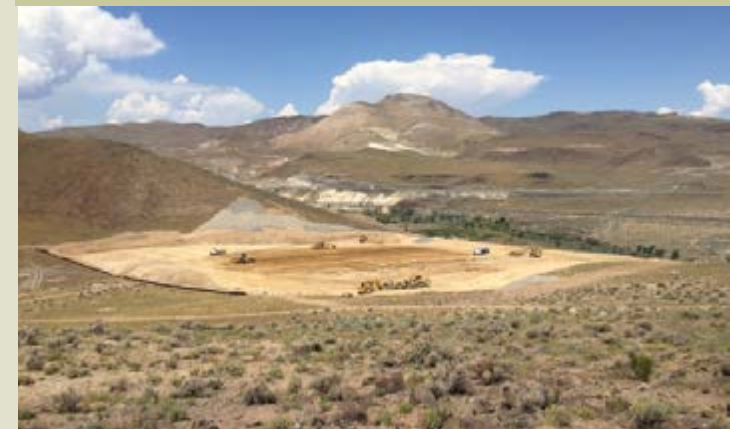
Construction of the Sierra Biofuels facility outside Reno
