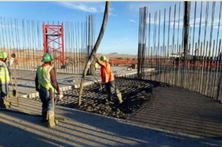
Construction of the Crescent Dunes solar project in Nye County.
