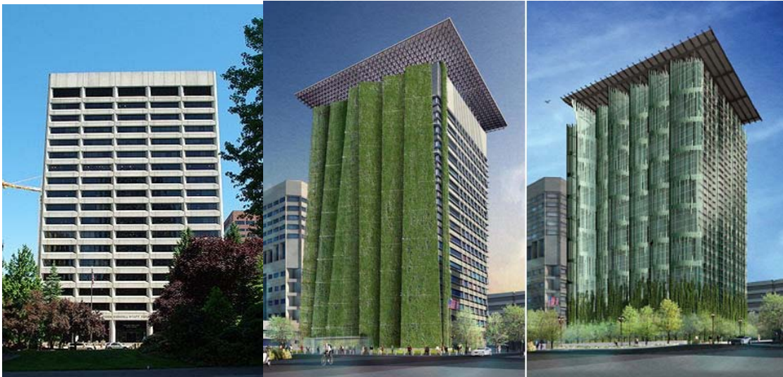
The current building, green wall, and final design of the Green-Wyatt Federal Building in Portland, OR
