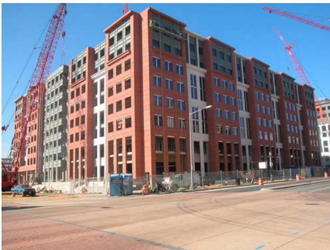
U.S. Department of Transportation Headquarters, Washington, D.C.
