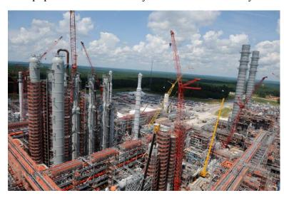
Southern's Kemper Project in Progress: "The Kemper plant will use two commercial-scale TRIG™ units to gasify lignite (low-rank coal that is mined next to the facility) to produce syngas. After the syngas leaves the gasifiers, it will be cleaned and used as fuel for two combined-cycle power generating units with a net output of 582-megawatts of electricity." Global CCS Institute Status of CCS.
