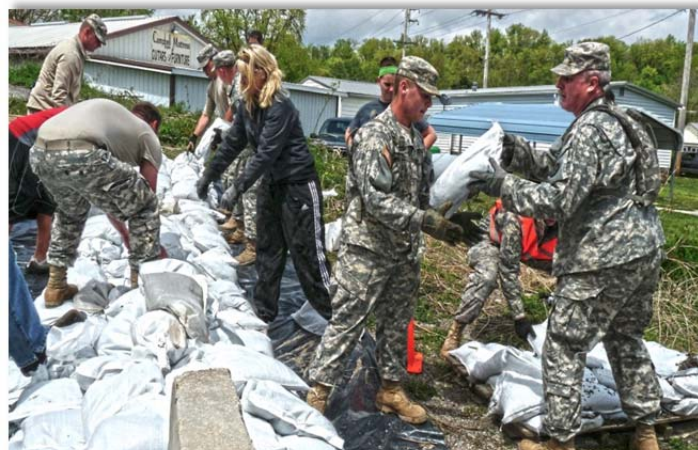
Soldiers of the 1140th Engineer Battalion, civilian first responders, and local residents work quickly to build a three-foot sandbag wall to prevent possible flood waters from closing a Missouri highway intersection. (Photo by Michelle Queiser/Missouri National Guard)
