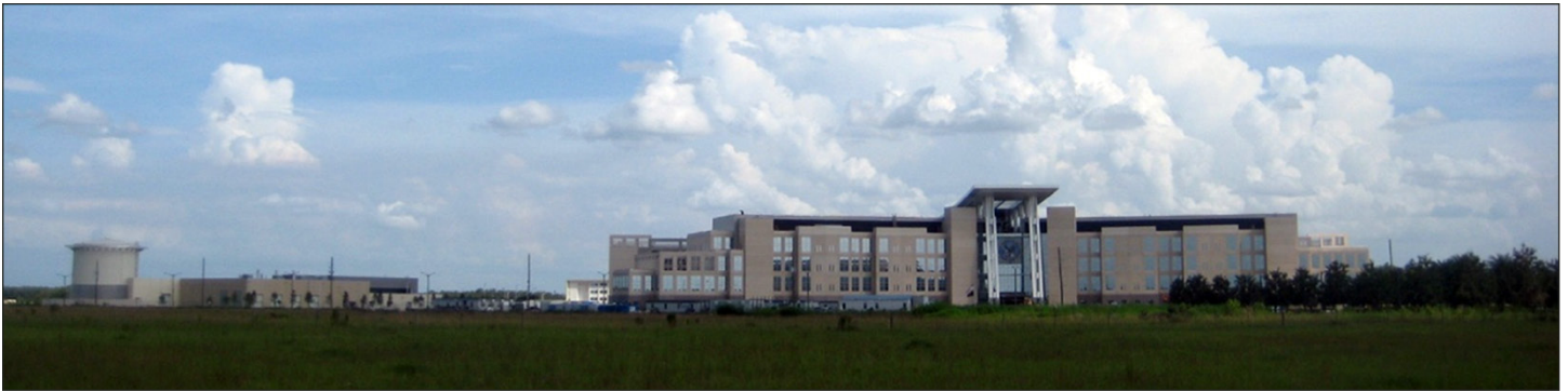
Figure 3: Current Site and Construction of the Orlando VA Medical Center Project
