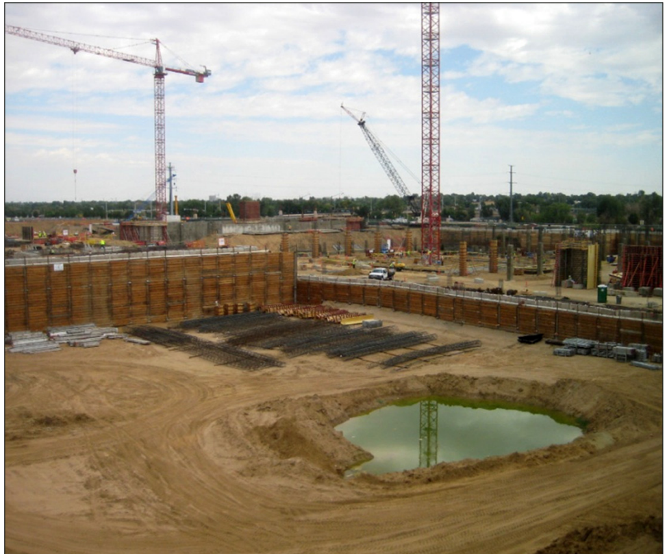
Figure 4: Underground Spring Located at the Denver VA Project Site
