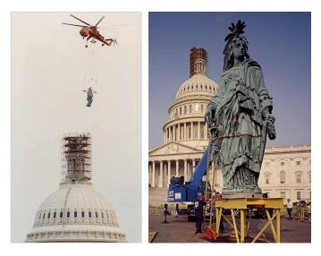
The bronze statue was removed by helicopter to the East Front plaza for restoration in 1993. Surface corrosion and discoloration of caulk in the seams were the most visible signs of its exposure to the elements for over a century.
