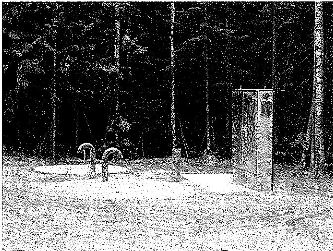
A sanitary lift station, part of a wastewater collection system. Typical of the type of project components constructed under the Section 219 Program.
