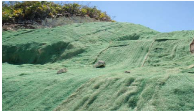
Terraces and geotextile
