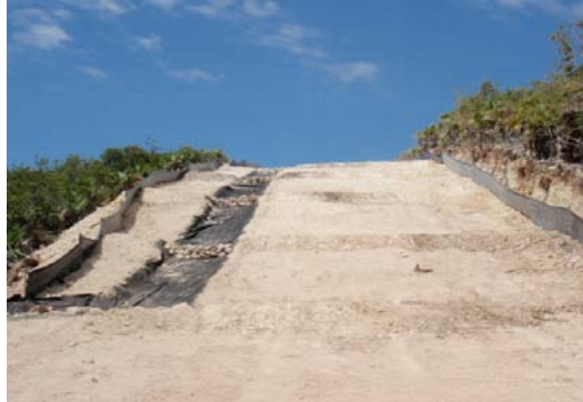
Longitudinal/transversal furrows and velocity dissipation devices
