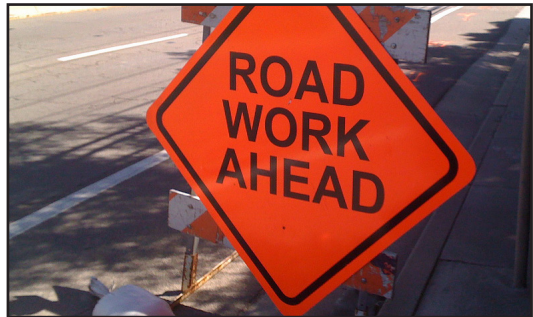
The Paramount Boulevard overpass is now closed for construction
