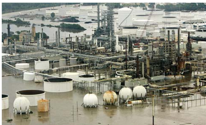
Hurricane Katrina damaged oil infrastructure throughout the Gulf.
