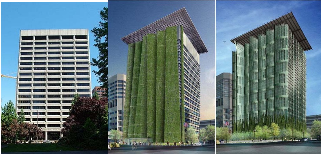
The current building, green wall, and final design of the Green-Wyatt Federal Building in Portland, OR
