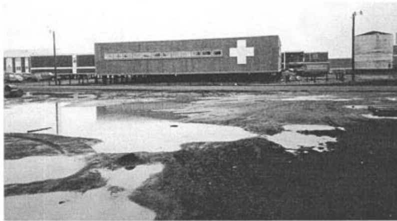
This hospital in Barrow, Alaska has been on the IHS facility list since 1991 and is in desperate need of replacement.
