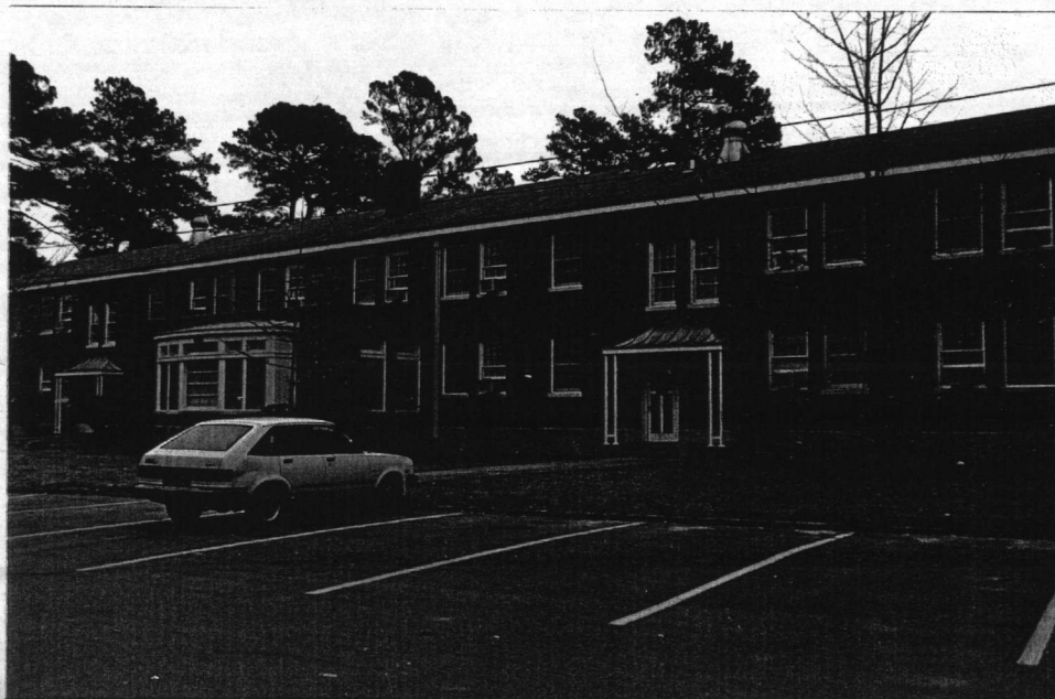
BOQ BUILDING 2603 - REAR VIEW
