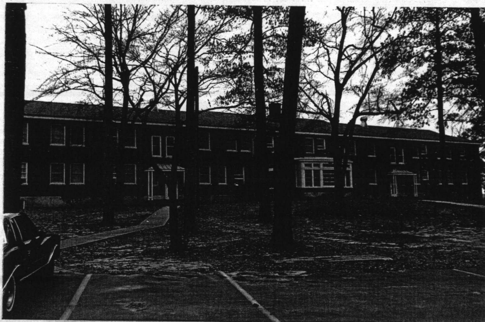
BOQ BUILDING 2607 - REAR VIEW
