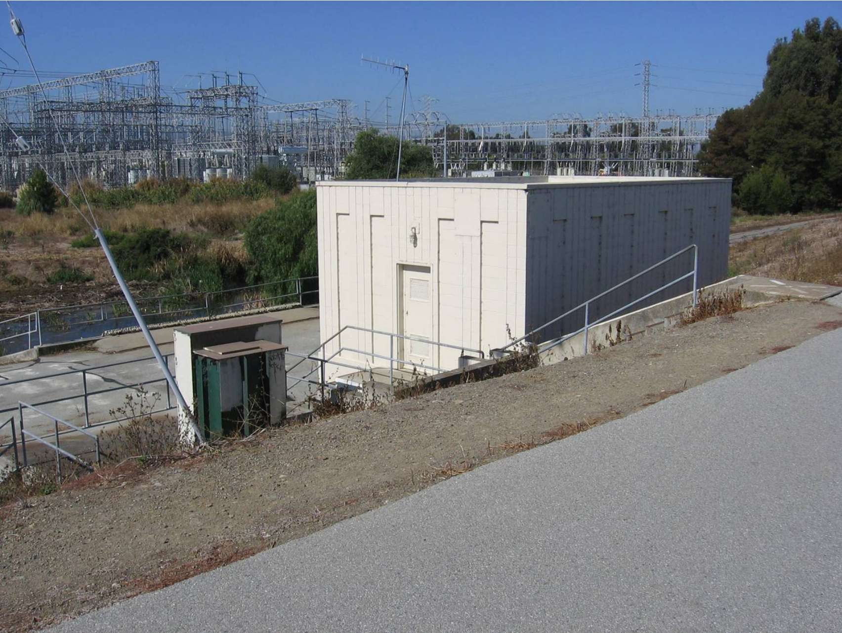
Poplar Pump Station Exterior
