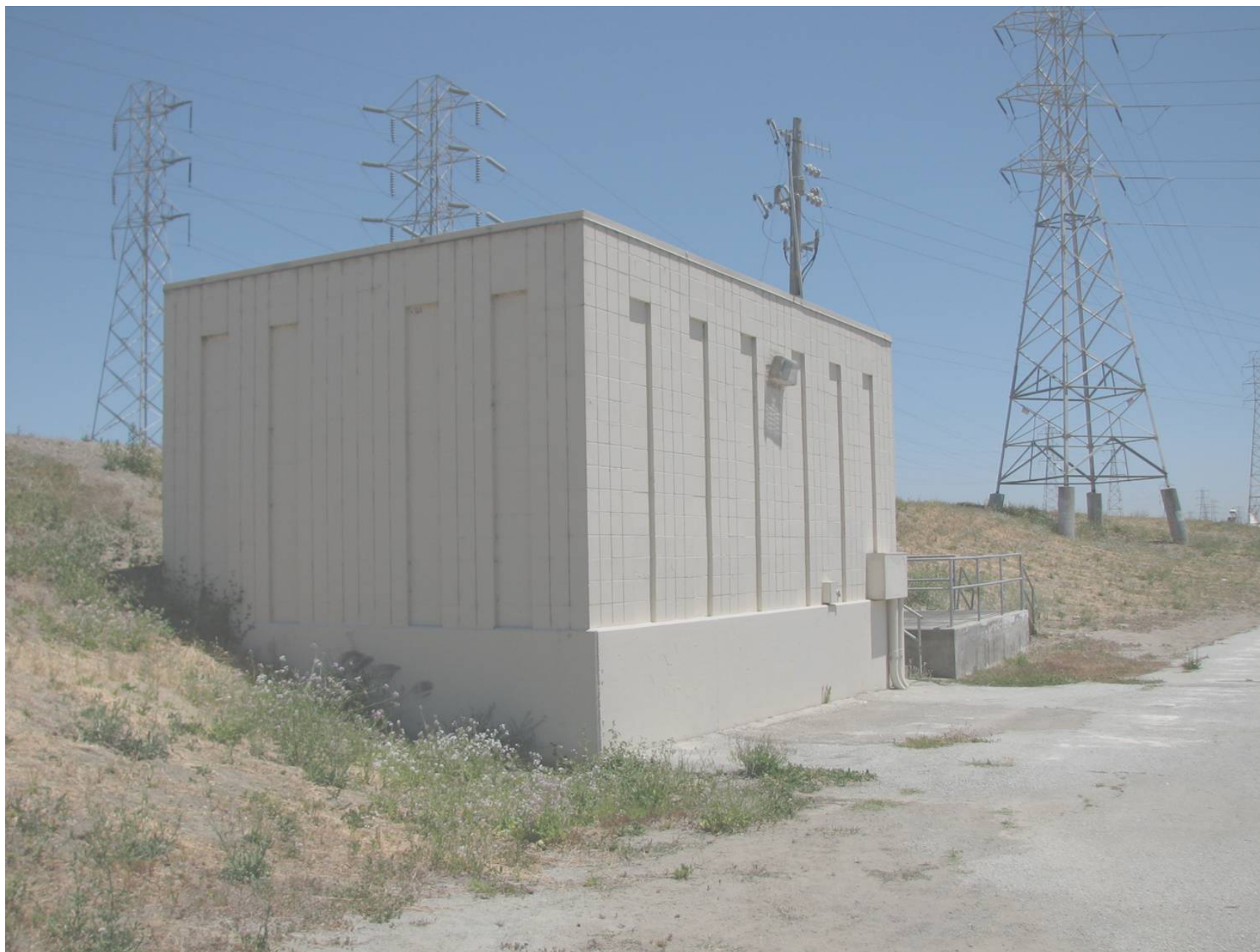
Poplar Pump Station Exterior
