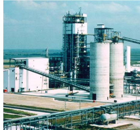
The Tampa Electric Coal Gasification Combined Cycle Plant
