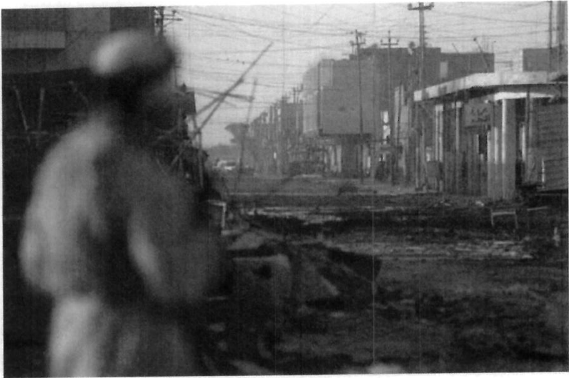
Figure 26 Low hanging wires located throughout the ITO
