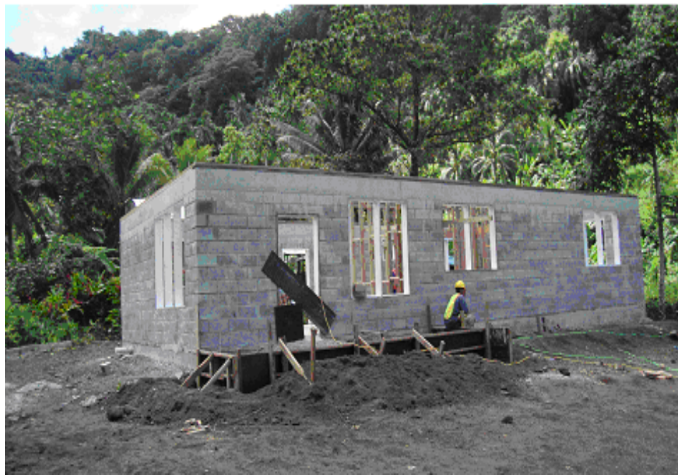
Figure 8. FEMA Home Under Construction in American Samoa
