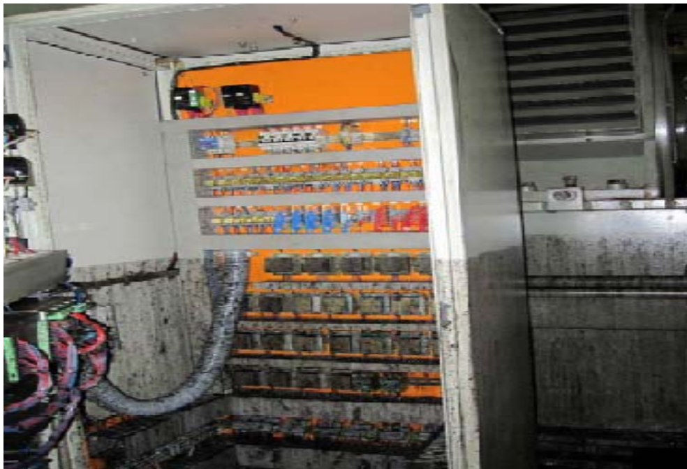
Figure 6. Destroyed Generator at Satala Power Plant
