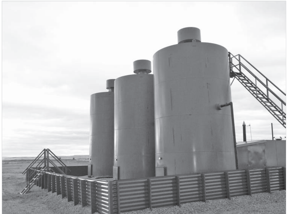
Figure 2: Oil Tanks in Carlsbad, New Mexico
