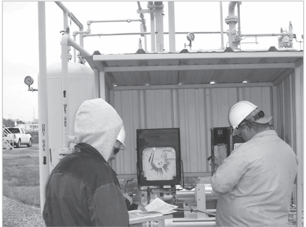
Figure 6: OEMM Inspectors Witnessing a Calibration of an Orifice Meter Associated With a Chart Recorder at a Land-Based Meter Location
